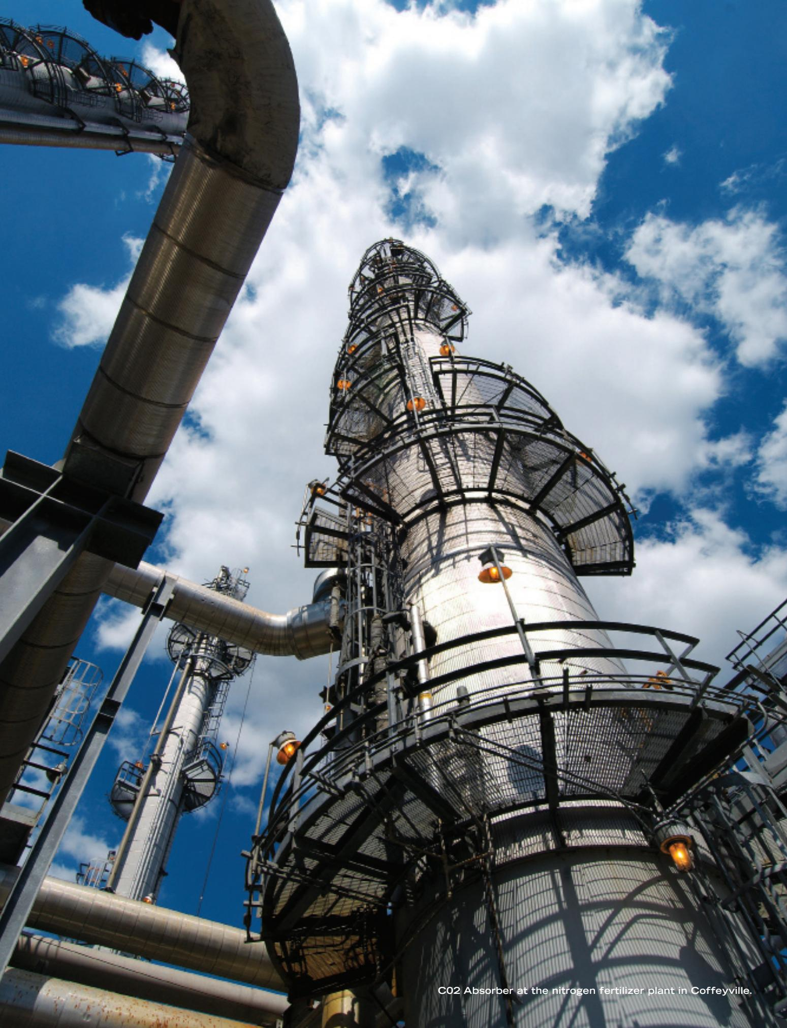
CO<sub>2</sub> Absorber at the nitrogen fertilizer plant in Coffeyville.
